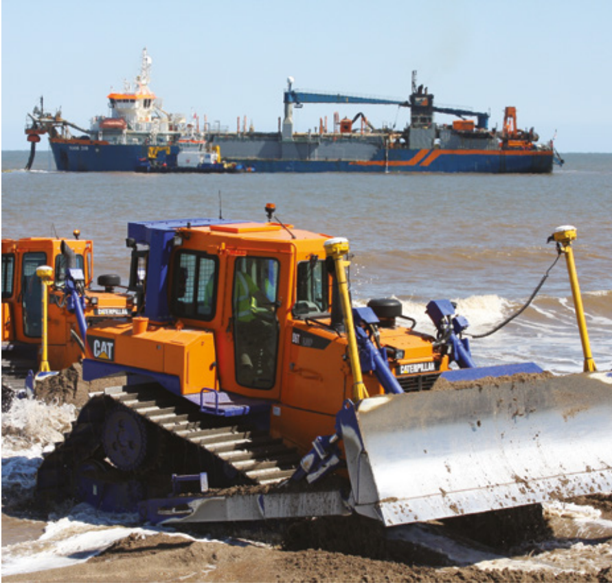
IMAGE SUPPLIED BY VAN OORD UK LTD
