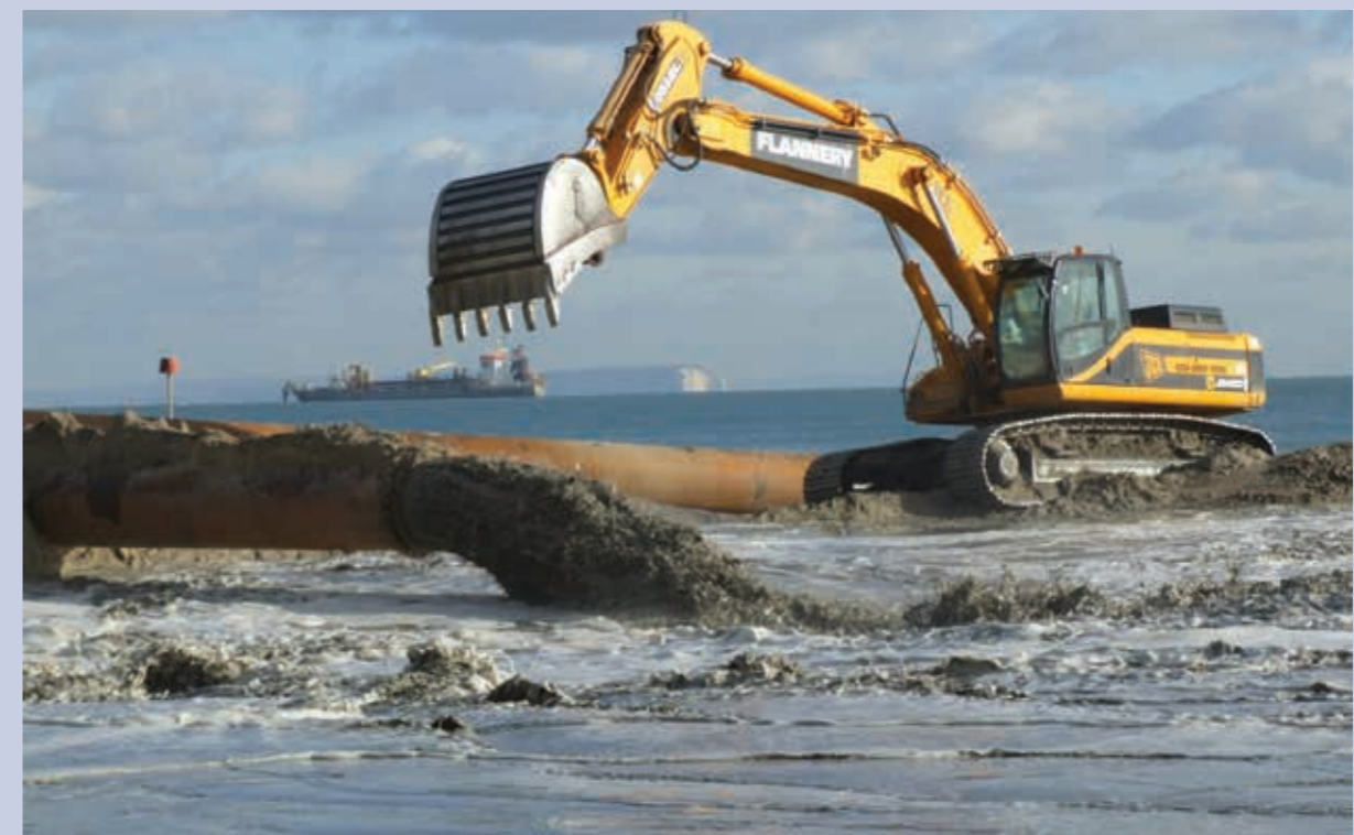
FIGURE 15: Since 1999, over 16 million tonnes of marine sand and gravel has been used for beach replenishment projects such as this example, taking place at Bournemouth, Dorset.
